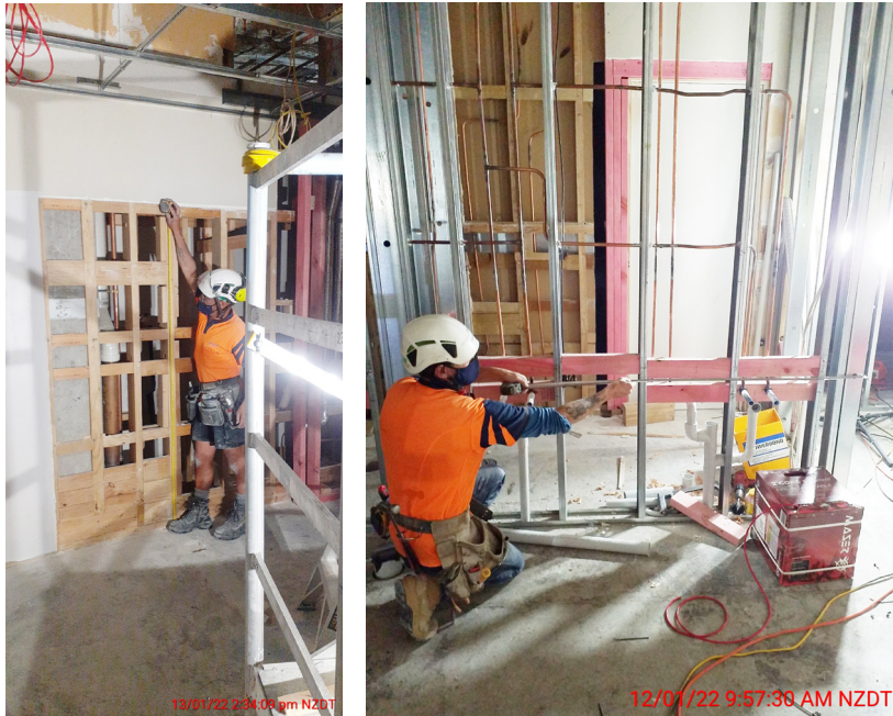
The new change rooms taking shape.
