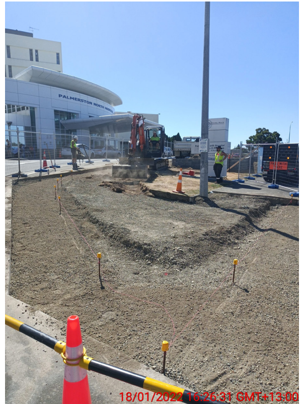
SPIRE construction continues
