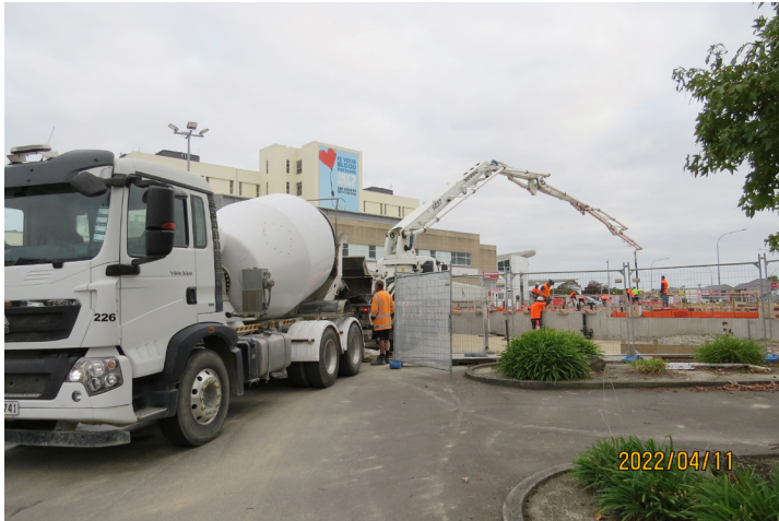
Foundation being laid for MAPU-EDOA facility.
