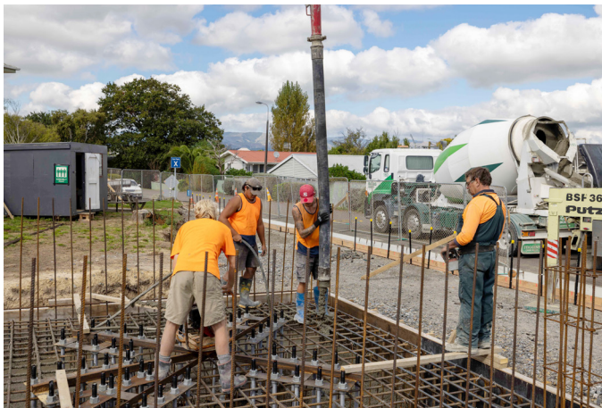
The concrete pour (35 cubic metres) was one of the last steps in completing the foundation pad for the new oxygen tank.
