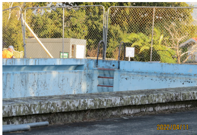
The old swimming pool is to be removed to make way for our water farm.
