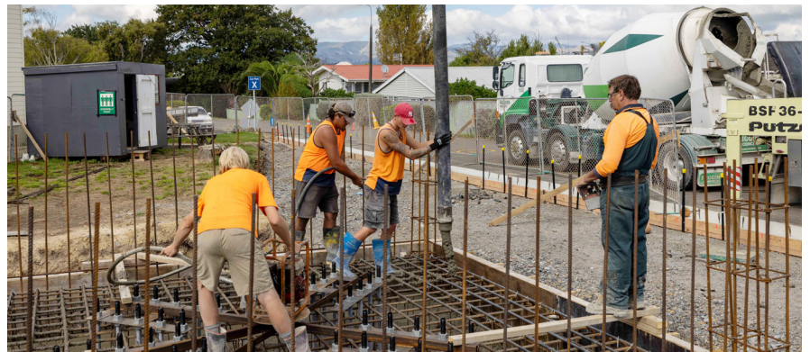
Foundation pad laid in readiness for new oxygen tank.
