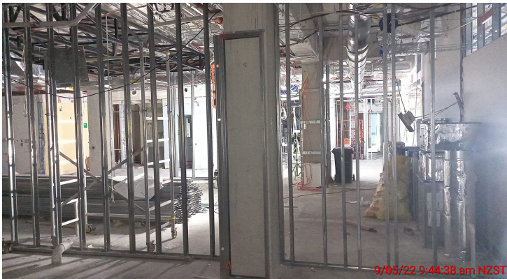
Rooms framing within SPIRE stage 1 going up.
