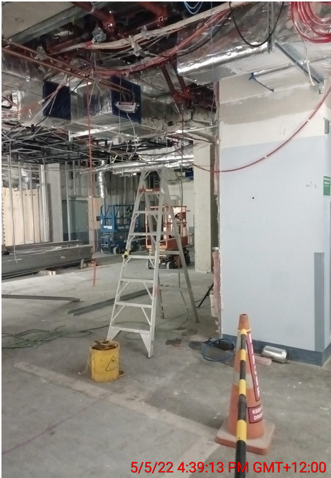
Work to install services throughout the ceiling space progressing well.
