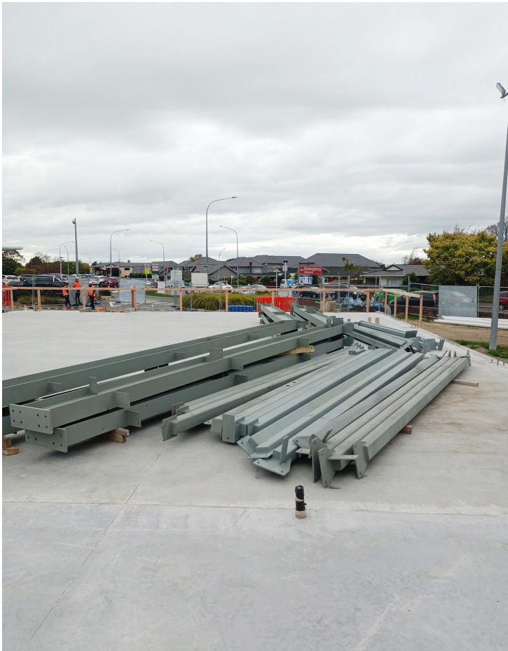
Foundations finished and steel framing arrives on site.
