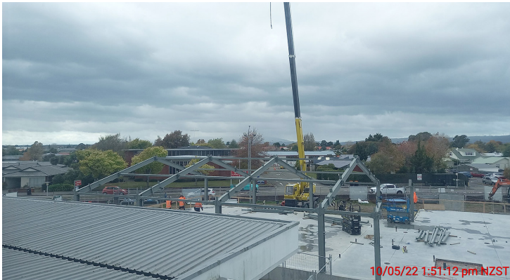
MAPU & EDOA foundation complete and steel portal frame being erected.
