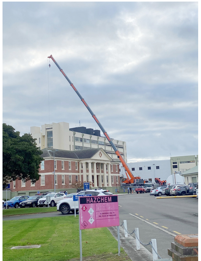
Scaffolding and materials for SPIRE craned in.
