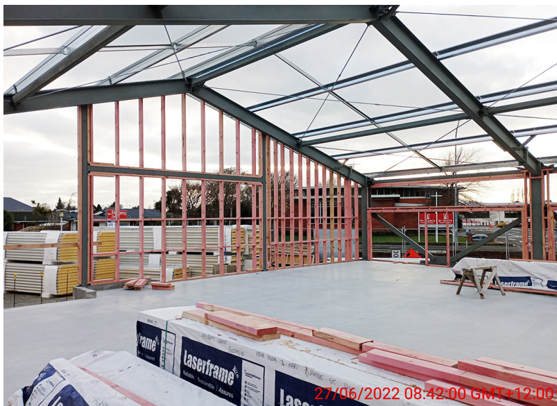
MAPU/EOA structure up, and framing underway.
