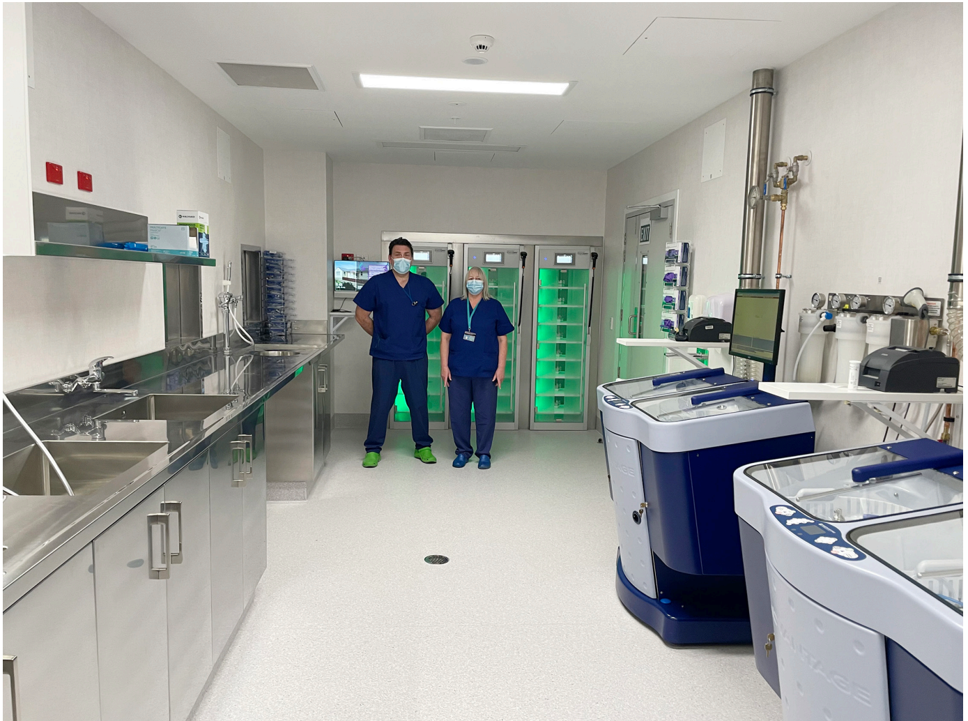
Next, the medivators are installed, then the drying cabinets.
