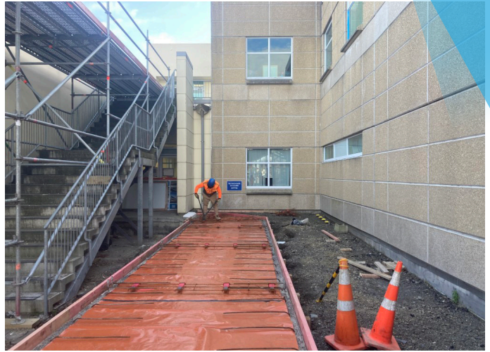
Link corridor to hospital under development.
