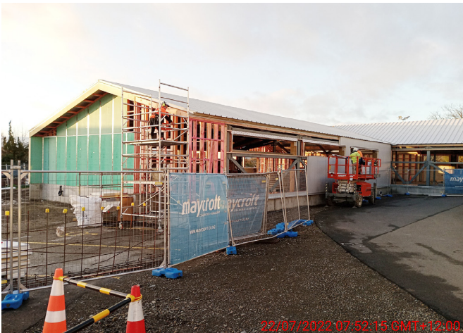
MAPU/EDOA unit well underway.
