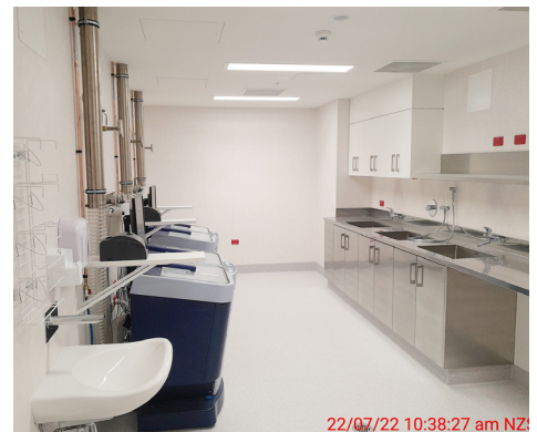
Then the sink and floor finishes.
