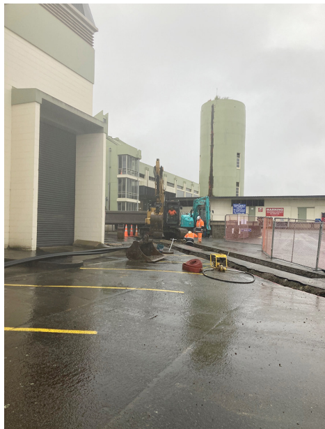
Trenches made for the new medical oxygen pipework.
