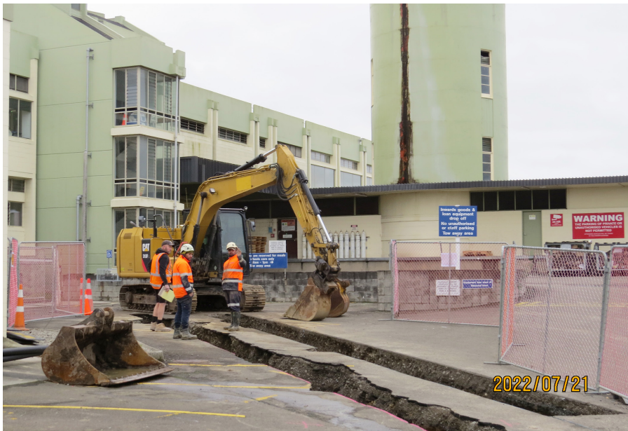
Inspection of work to date in progress.
