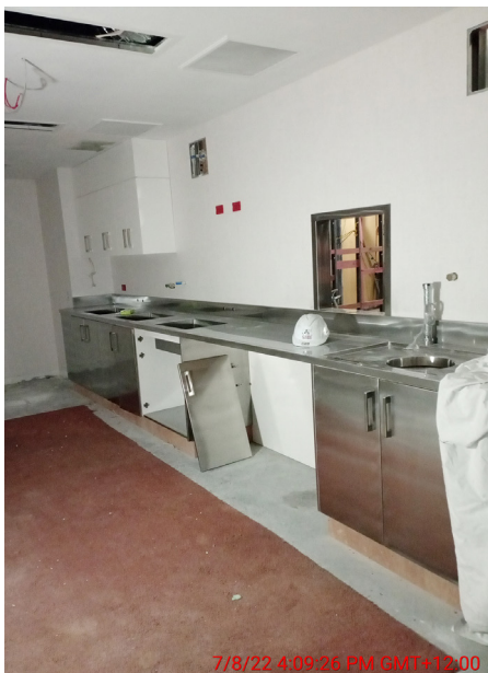
First the stainless-steel bench unit is built in.
