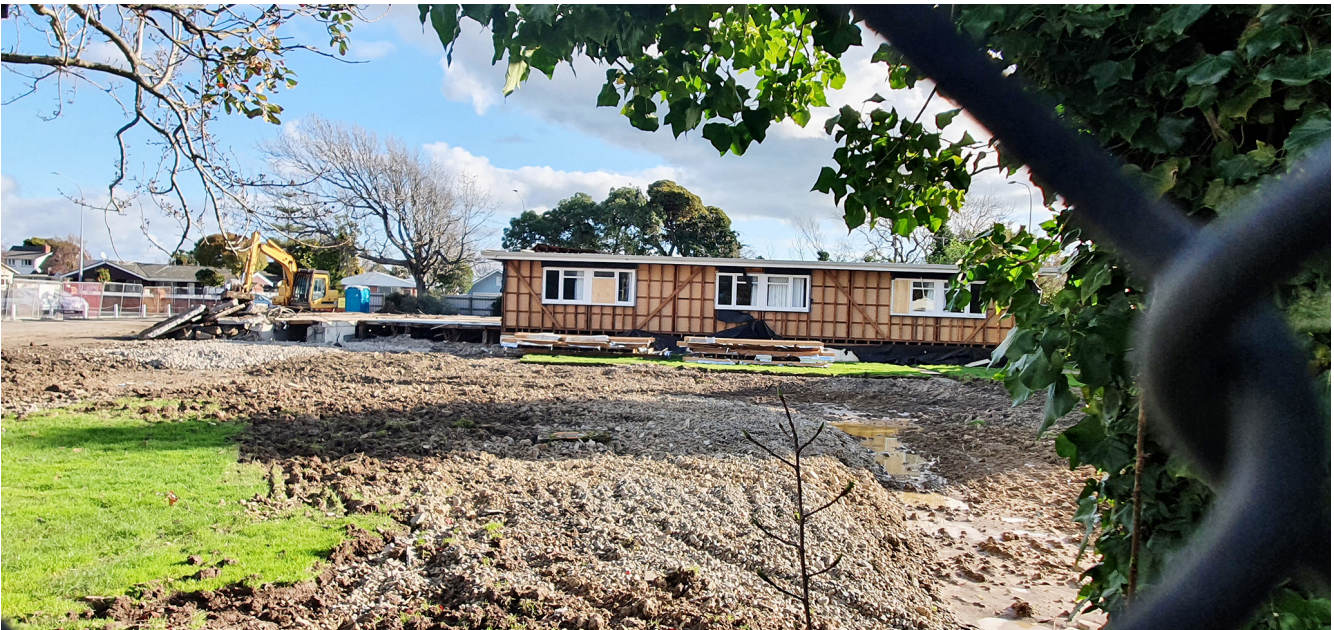
The last part of the building awaits disassembly.
