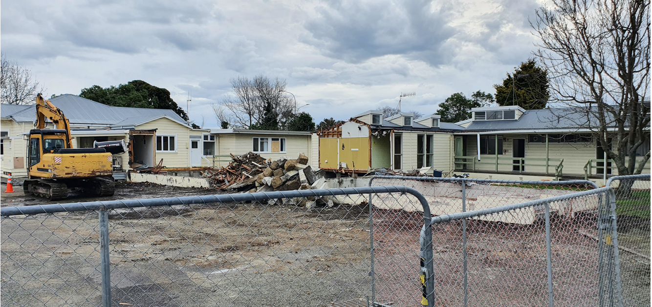
Deconstruction of Pullar Cottage commences.
