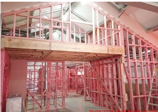
Internal framing of MAPU/EDOA underway.
