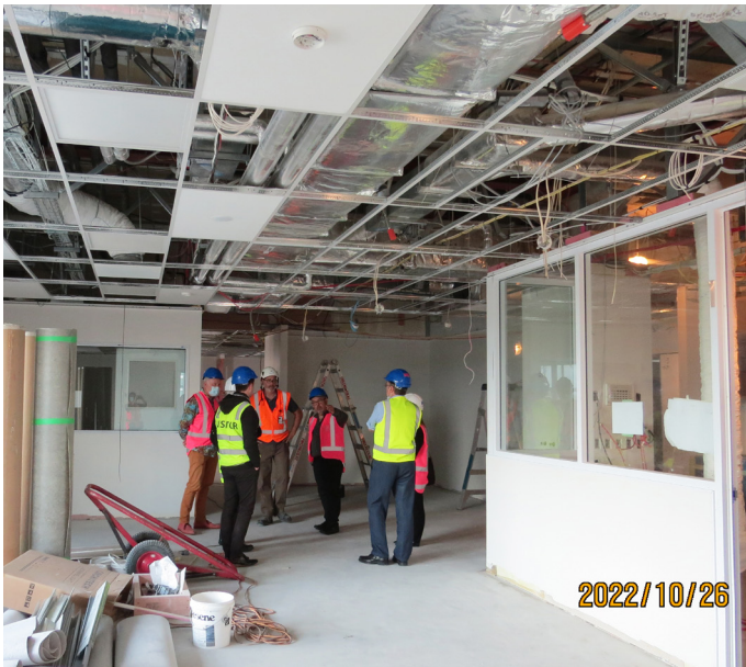
Day of surgery and recovery area painted and vinyl ready for laying.
