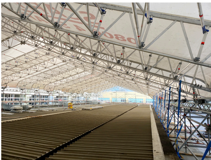
Roof work underway
