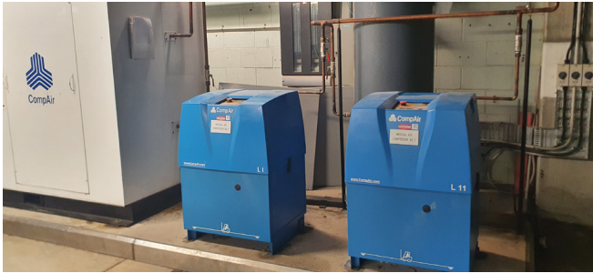
Current medical air system which does not have the capacity to meet our growing demand.
