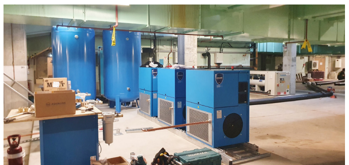
New medical air system being installed
