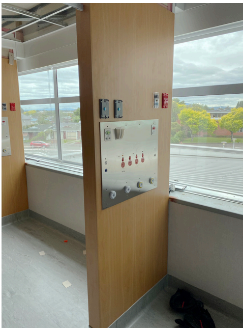
SPIRE Stage 1 nearing completion.
