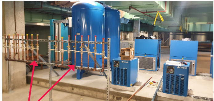
The new medical air system is taking shape, with the manifolds which regulate the air flow to the hospital being installed.
