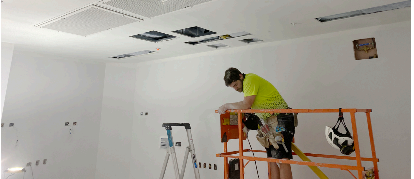
Finishing trades at work.
