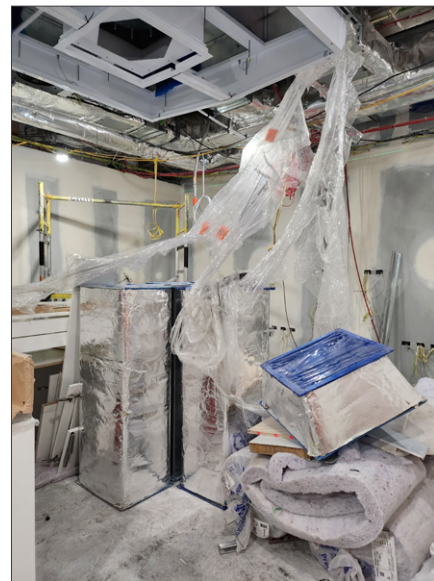
Demolition of old DOSA area underway.
