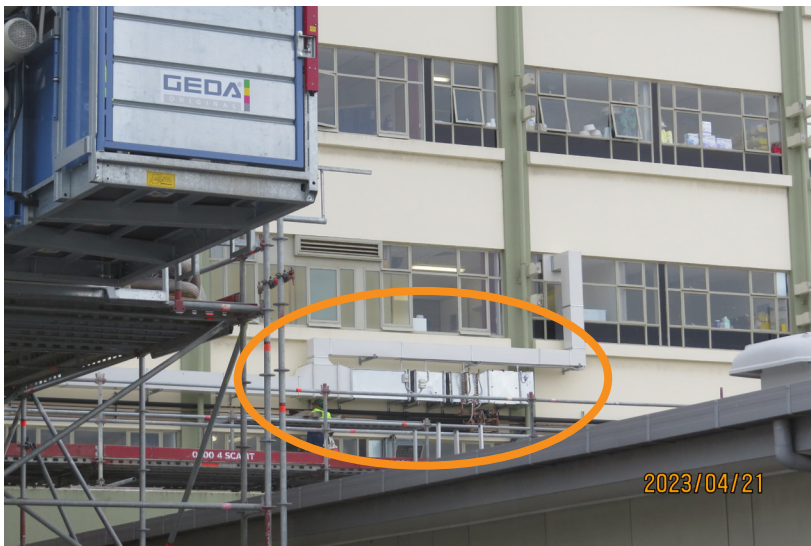
Pipework on the southern side of the building, brings air into the ward via the new ducting and air handling units.
