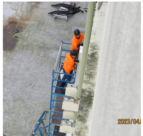
Pipework on the southern side of the building, brings air into the ward via the new ducting and air handling units.
