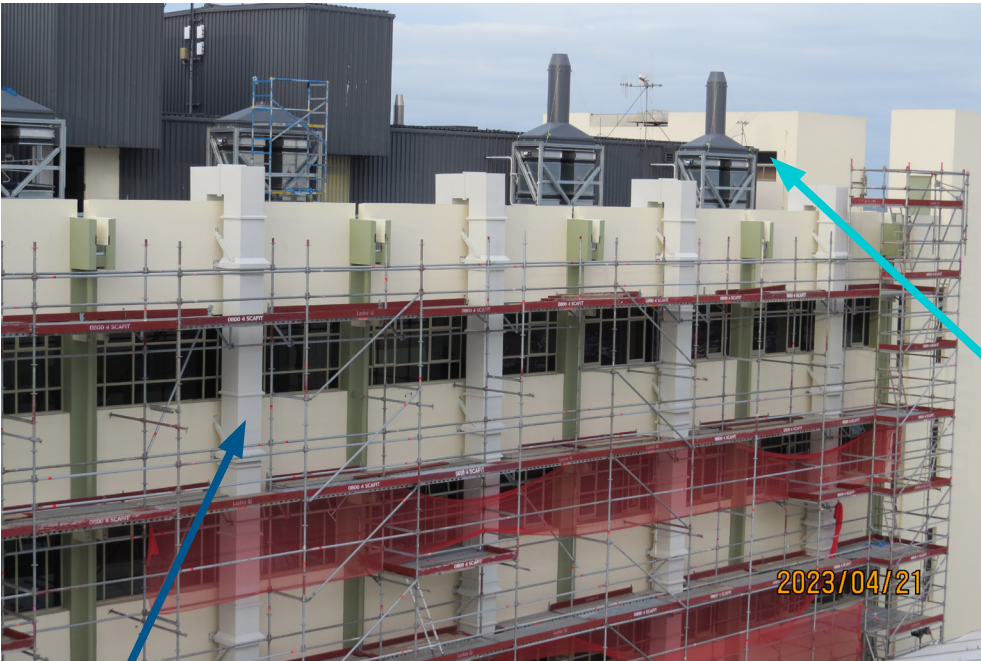
New ducting x 5 taking air up to HEPA filters.
