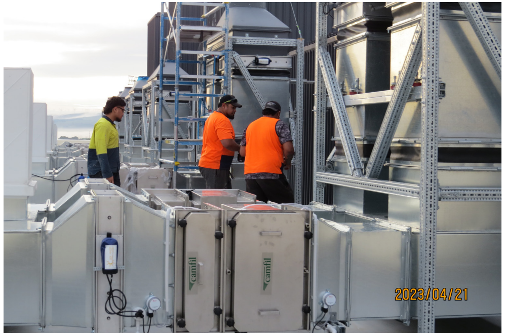
HEPA filters being installed.
